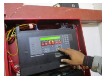
Fire detection control panel.JPG
