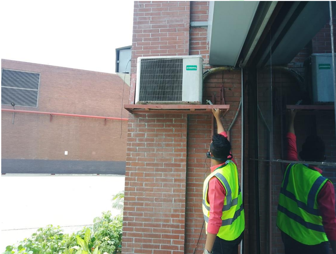
Figure: ODS leak test check
