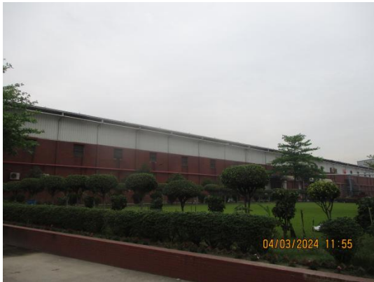
Facility Building -1.JPG
