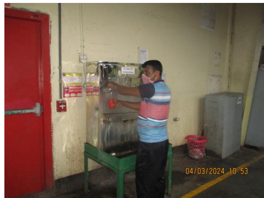
Drinking water facility.JPG
