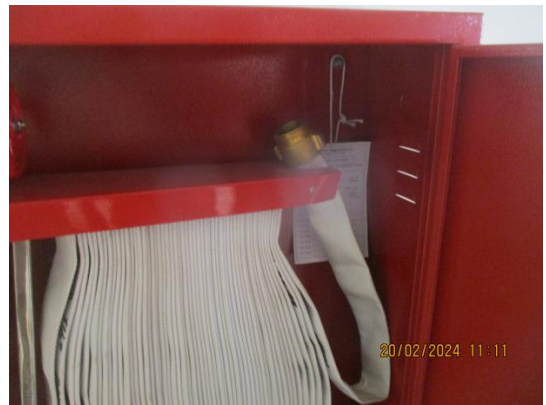
NC Photo-Fire hose without nozzle.JPG
