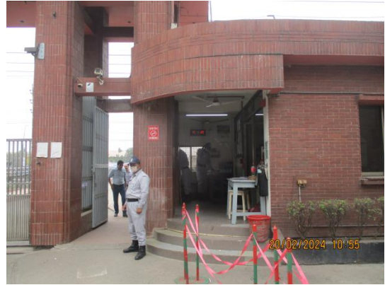
Security check room.JPG
